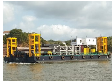
APCO GANGA 1 Jackup Barge M/s Apco Infratech Private Ltd.
