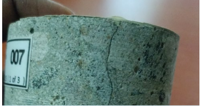
Verifying Post grouting Cracks are sealed after grouting
