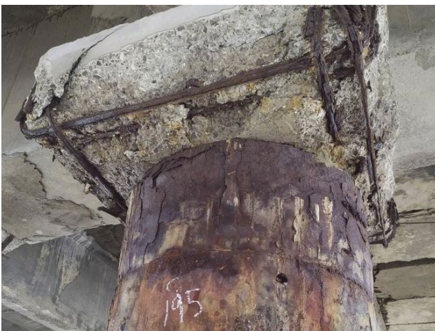
Corrosion of Sacrificial Liners & loss of strength in RCC elements
