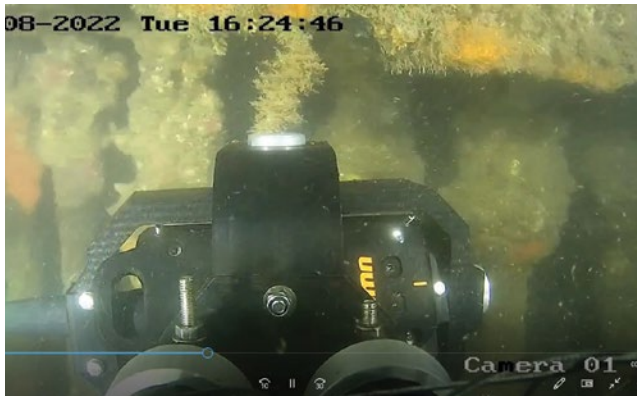
Underwater inspection for Piles
