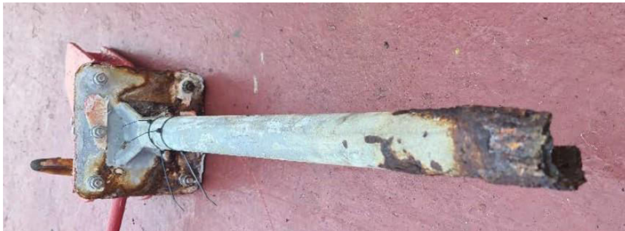
Figure 1: Photo of the rescue boat release hook support structure taken after the incident, showing significant deterioration of the post.
