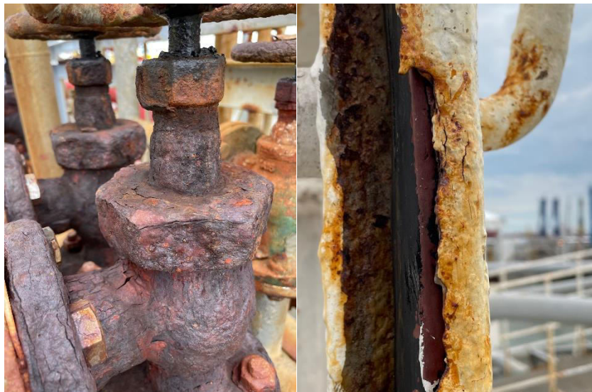
Figures 4 and 5: Typical on-deck condition (left) and watertight door (right).
