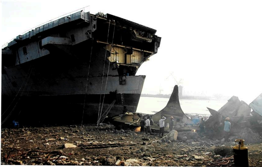
Around a quarter of the world's ships are recycled at Indian facilities, such as this shipbreaking yard in Darukhan
