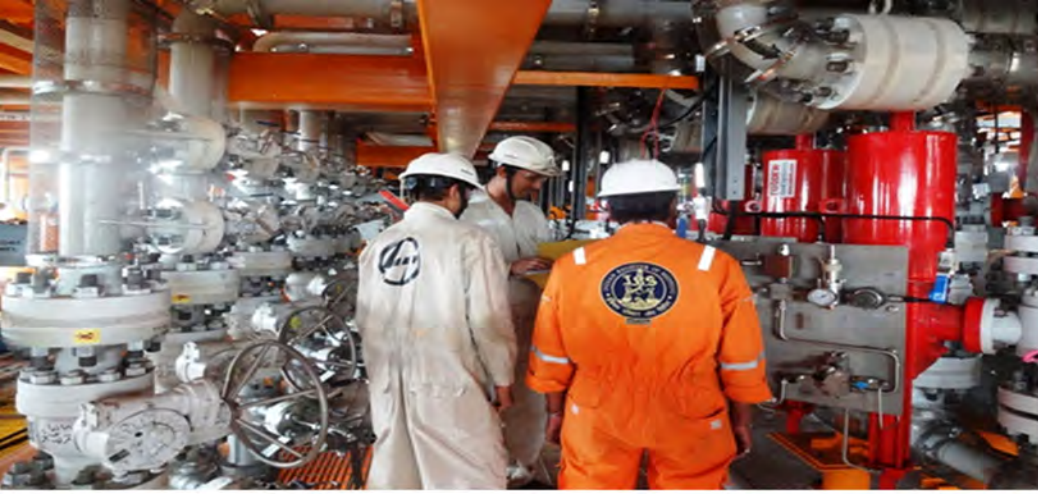
ISSPL Surveyors/Engineers checking the equipment and piping
